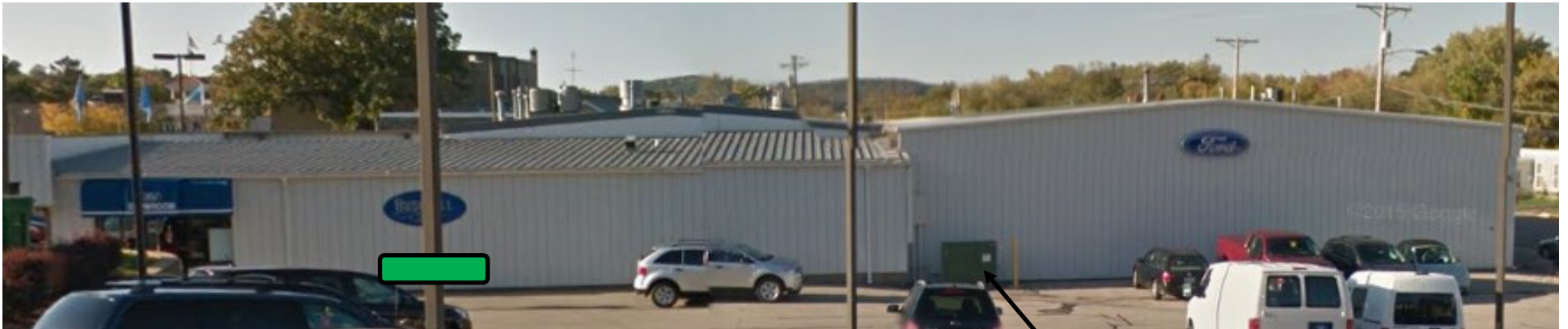
EV charging station Dual charger
